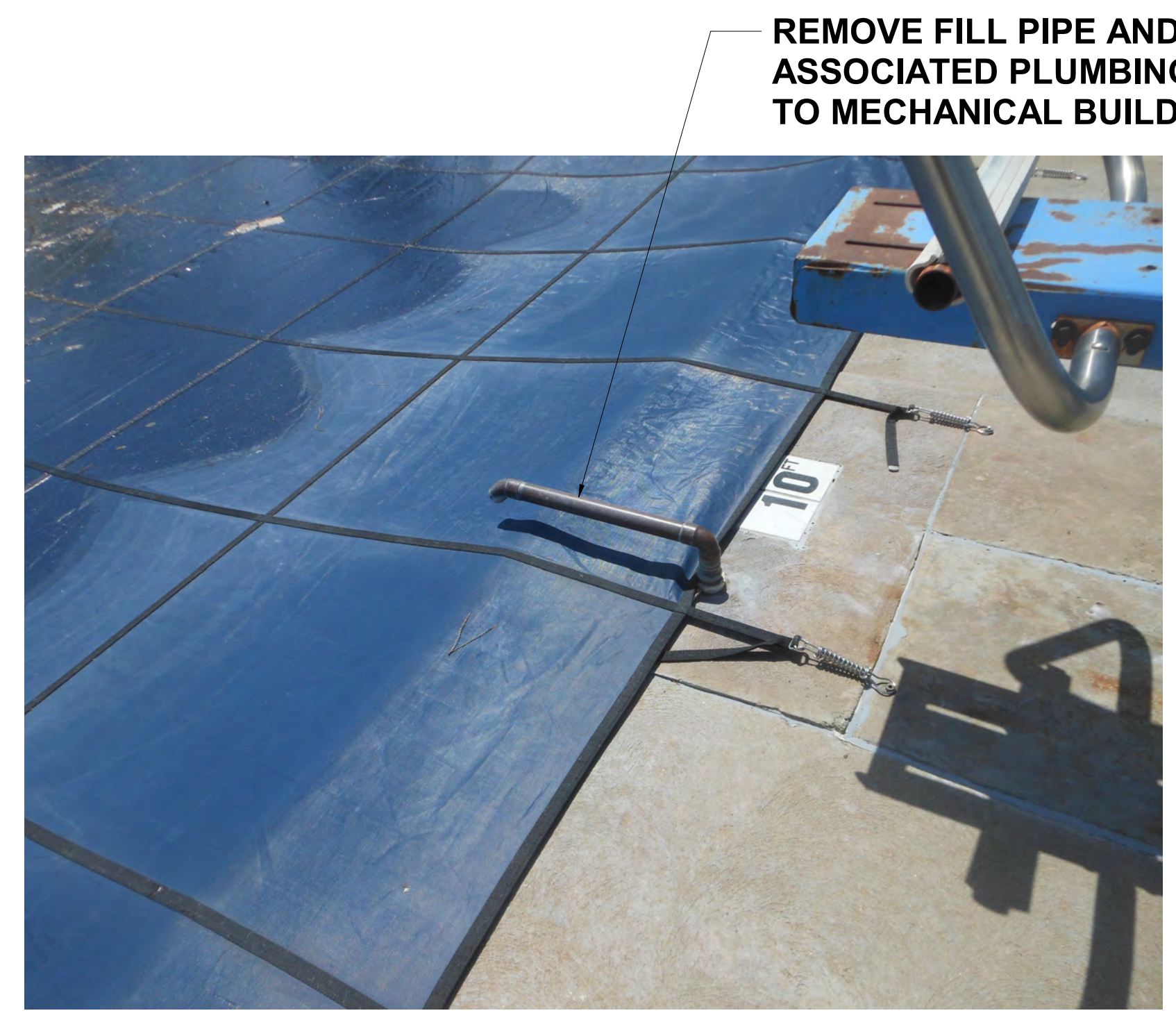
7 | EXISTING POOL FILL LINE DETAIL VIEW 1" = 10'-0"
